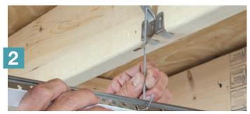
Suspend main beams with hanger wire or **NEW** QuickHang<sup>™</sup> hardware\* (shown above: QuickHang hooks and brackets)
